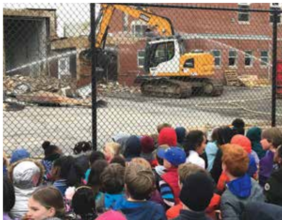
Field trip to witness Maury demolition
